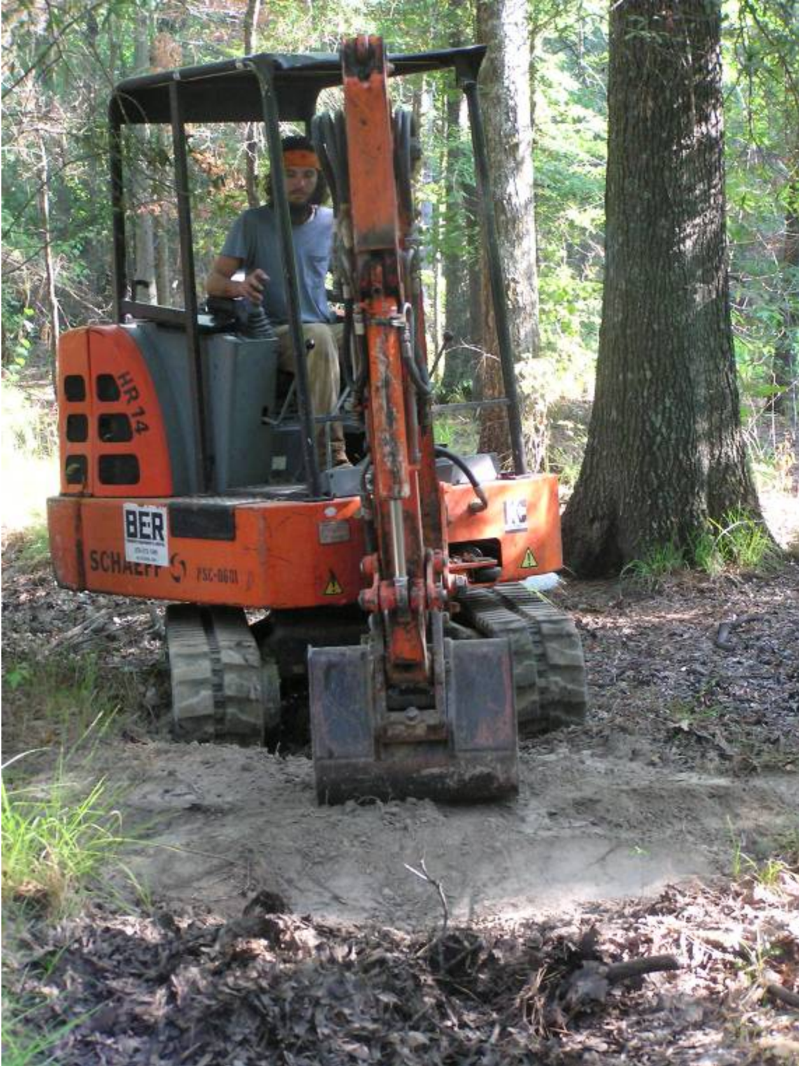
Fire Line Restoration
